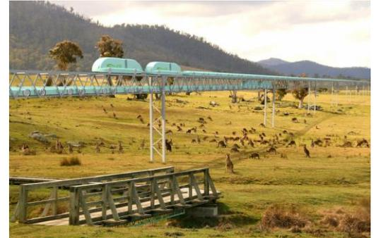
Unlike road or rail systems, because the system is elevated it can traverse mountains or other rough terrain and is not constrained by earthworks, embankments, sleepers and ballast, with minimal environmental impact at ground level.
